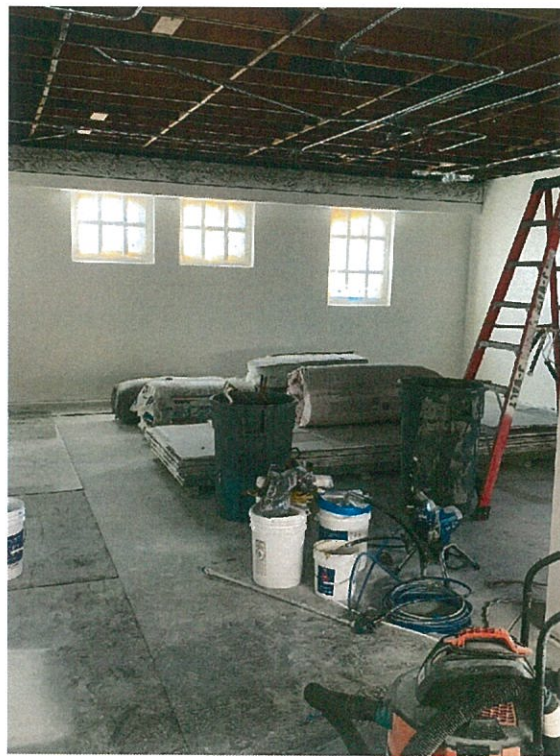
New Classroom View
