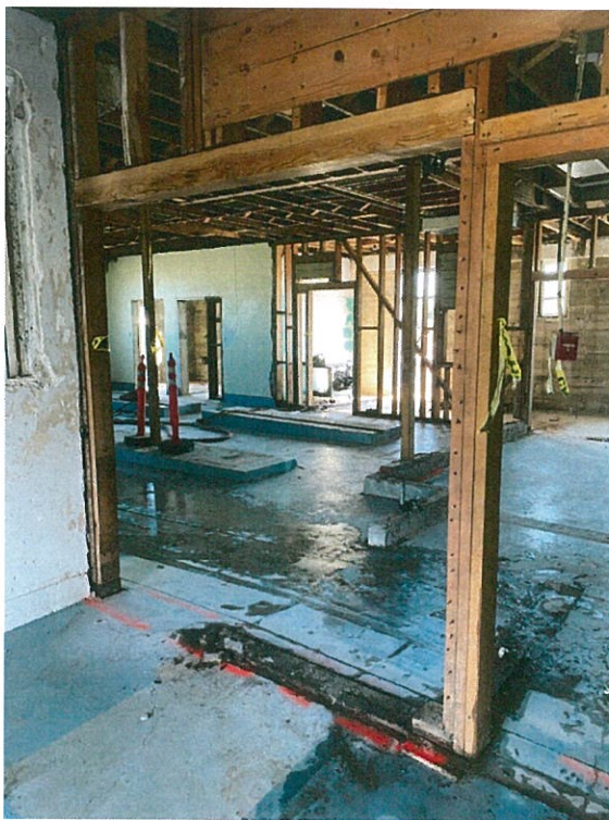
View of Locker Rm from Lobby Area
